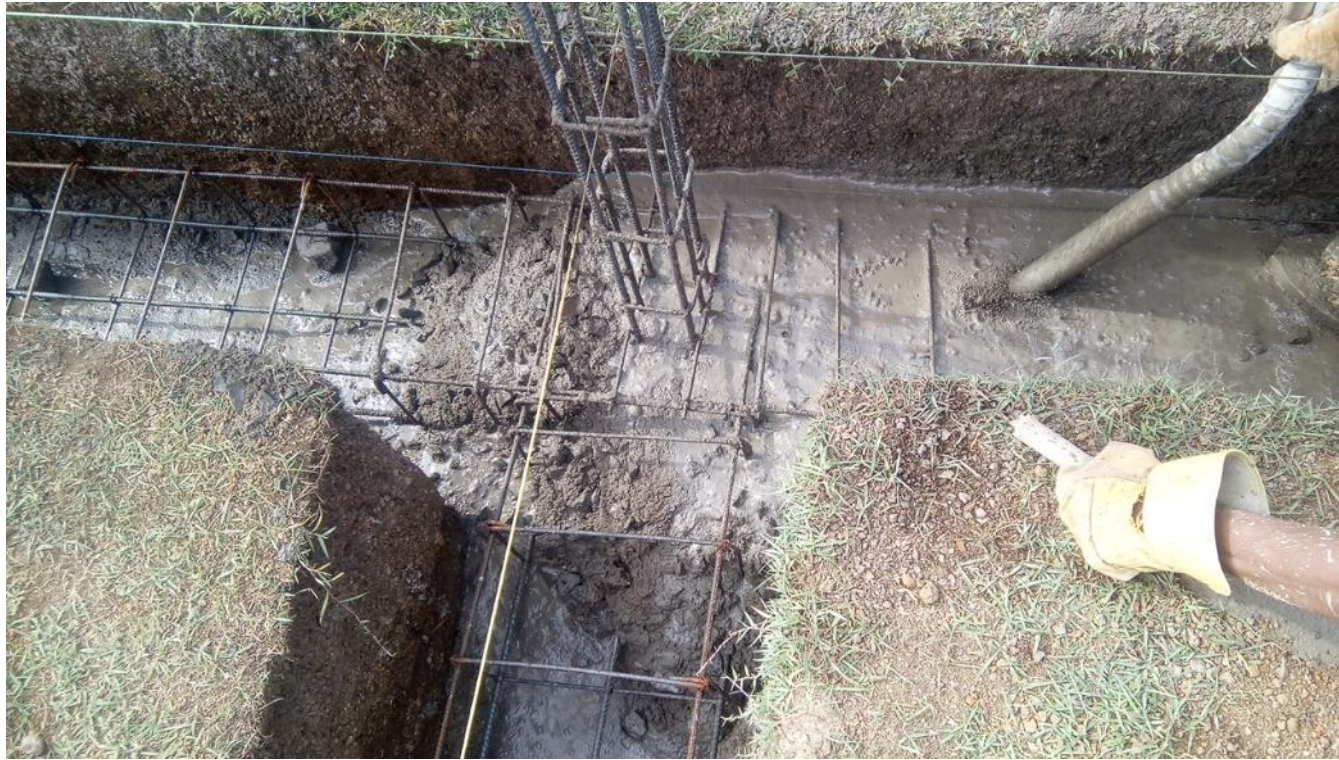
Vibrating the poured concrete
