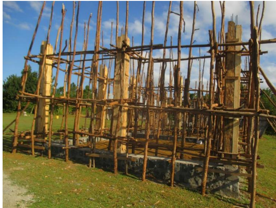
Surely they are ready and sure for pouring, tight to each other. Before pouring
