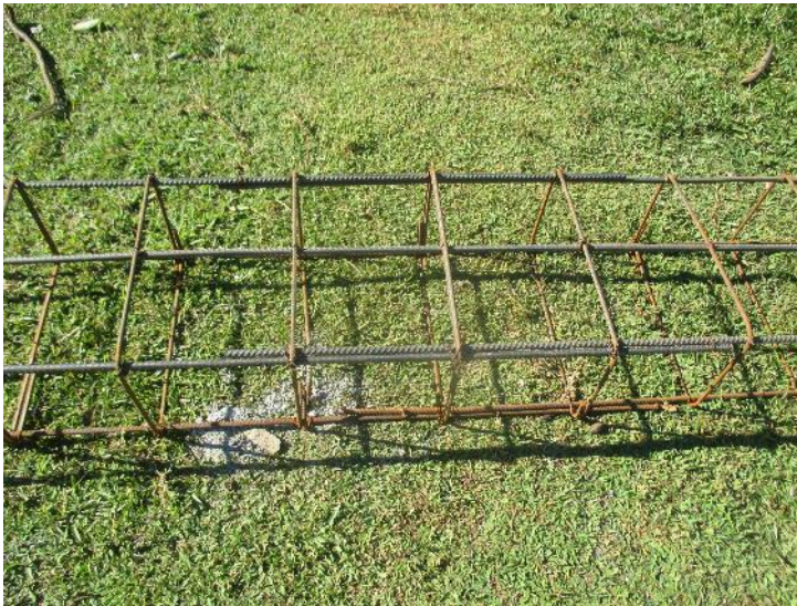
(Bottom view of ground beam's) Their Overlapping
