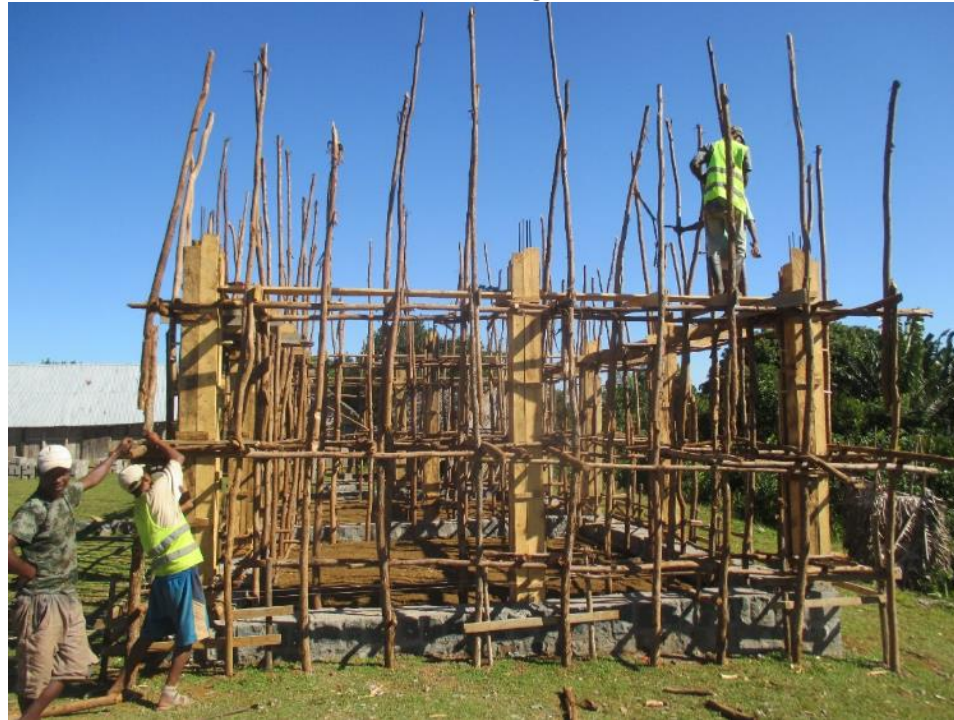
New used shuttering for column
