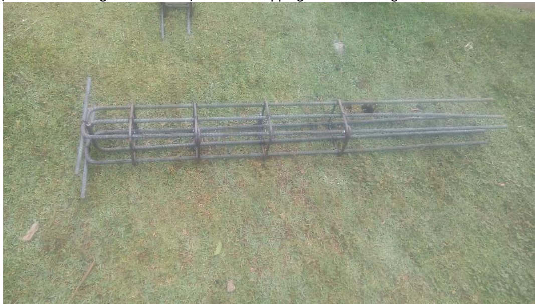
External Reinforcement of columns, 200*220mm of section
