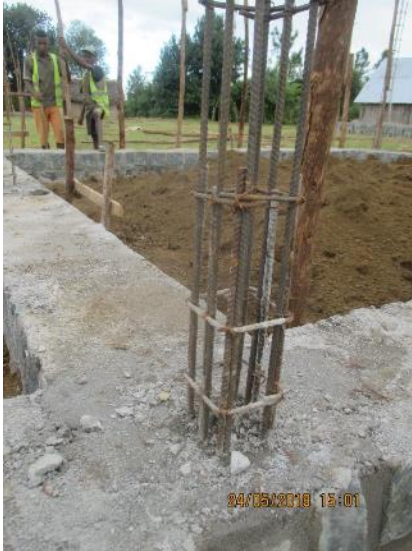
Reinforcement of column before pouring (Two identical schools) when it is poured in
