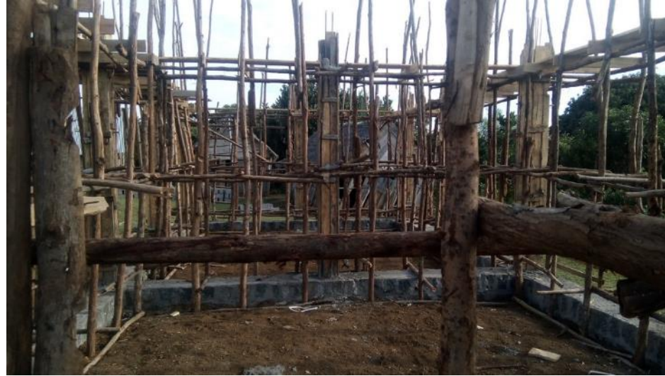
New used shuttering for column
