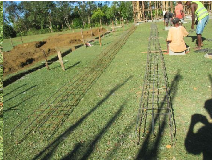
Longitudinal reinforcements in assembly or in preparation
