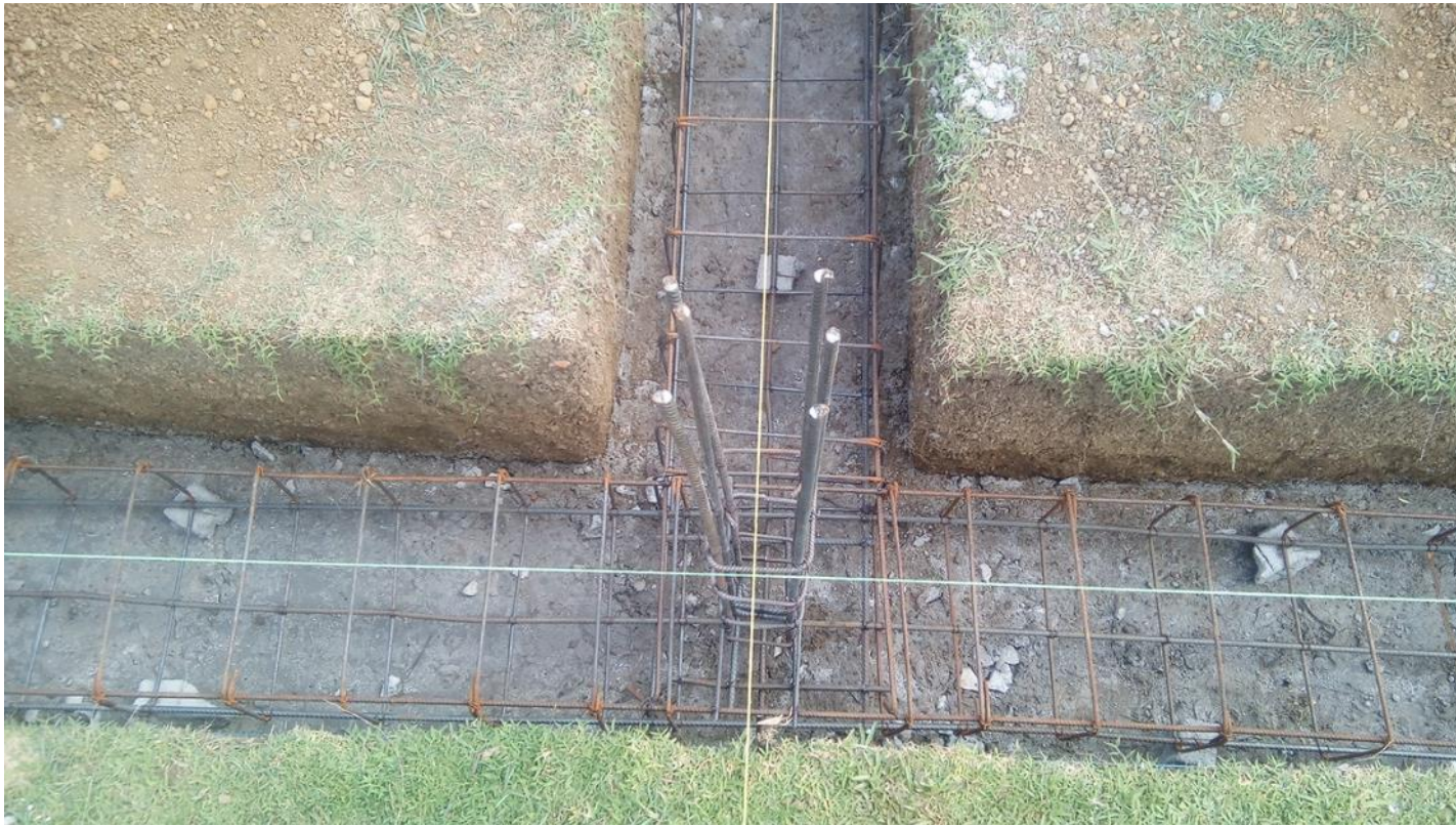
Connection between starter bars of column with the ground beams
