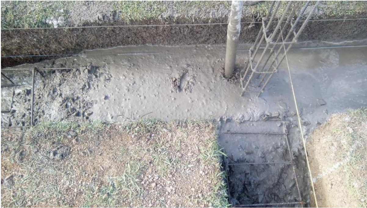
Pouring the junction of the foundation, middle of the reinforcement is respected
