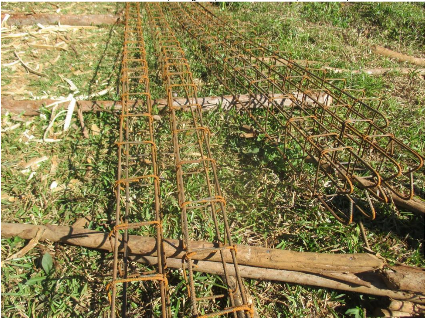
Prepared reinforcement of horizontal ring beams are already prepared in site. But the additional reinforcement are the missing things in them.
