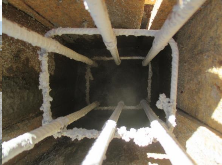
Reinforcement of column before pouring (Two identical schools) when it is poured in
