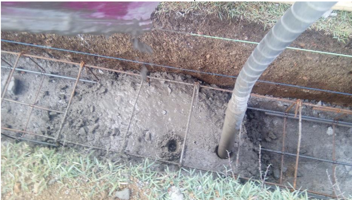
Poured concrete from the mixer was vibrated then
