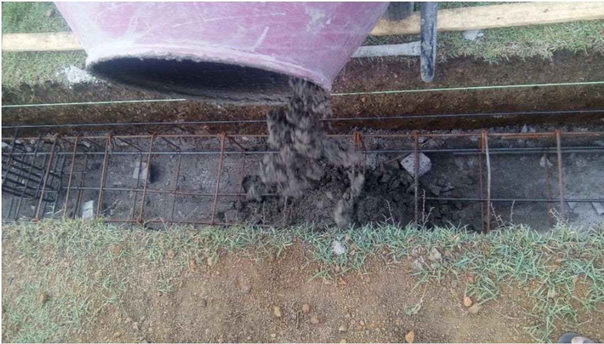
Mixer used in place
