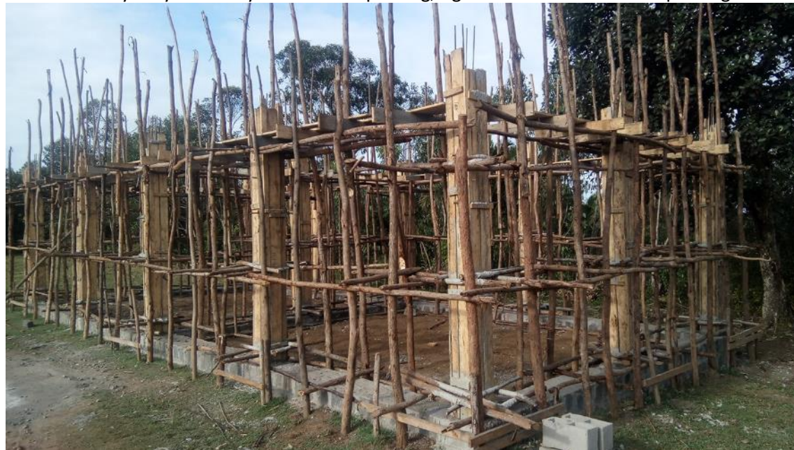
Scaffolding and shuttering of column after pouring
