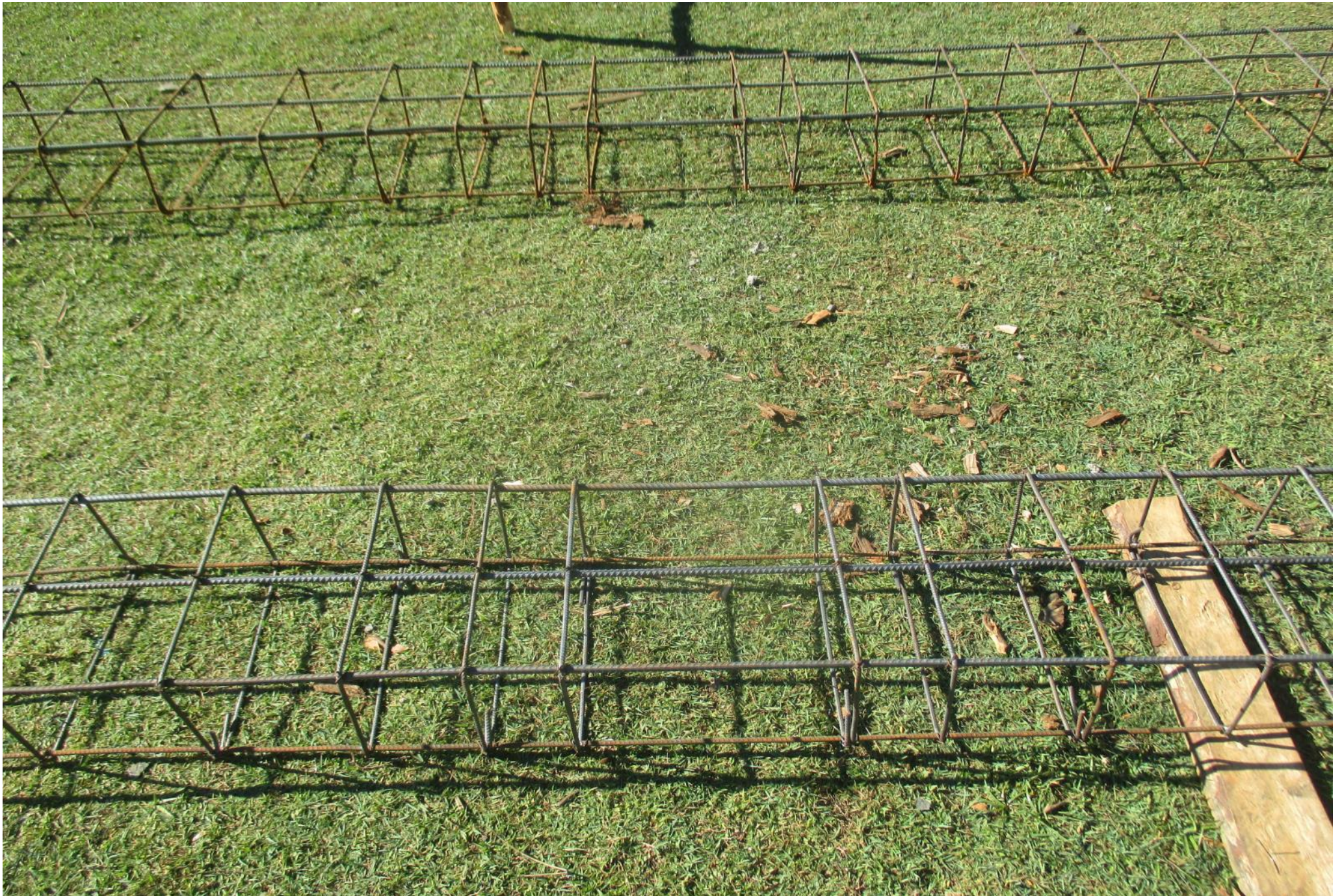
Reinforcement of ground beams in preparation (upset down situation)
