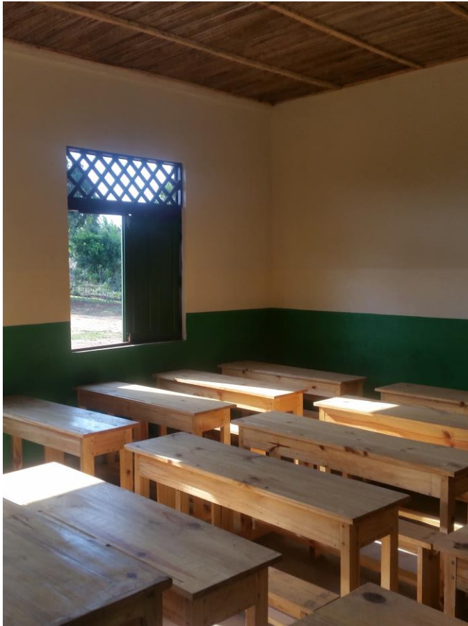
One of 6 new classrooms.
