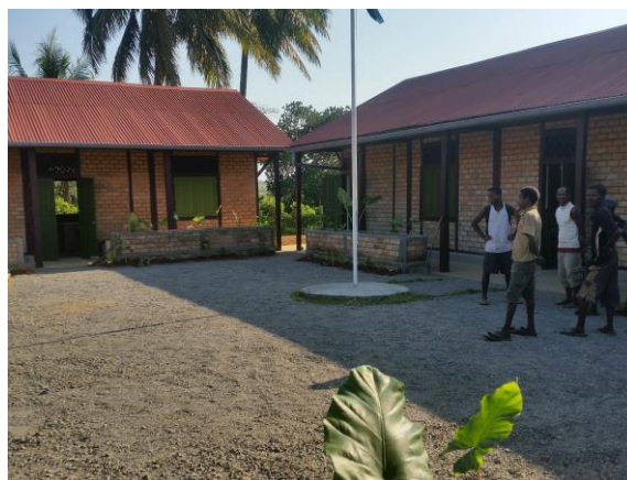
Central Courtyard and flagpole
