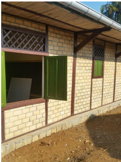
Rear Elevation of 1 classroom
