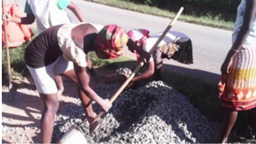
Preparing gravel required for work (above) & the initial state of infrastructure (below).
