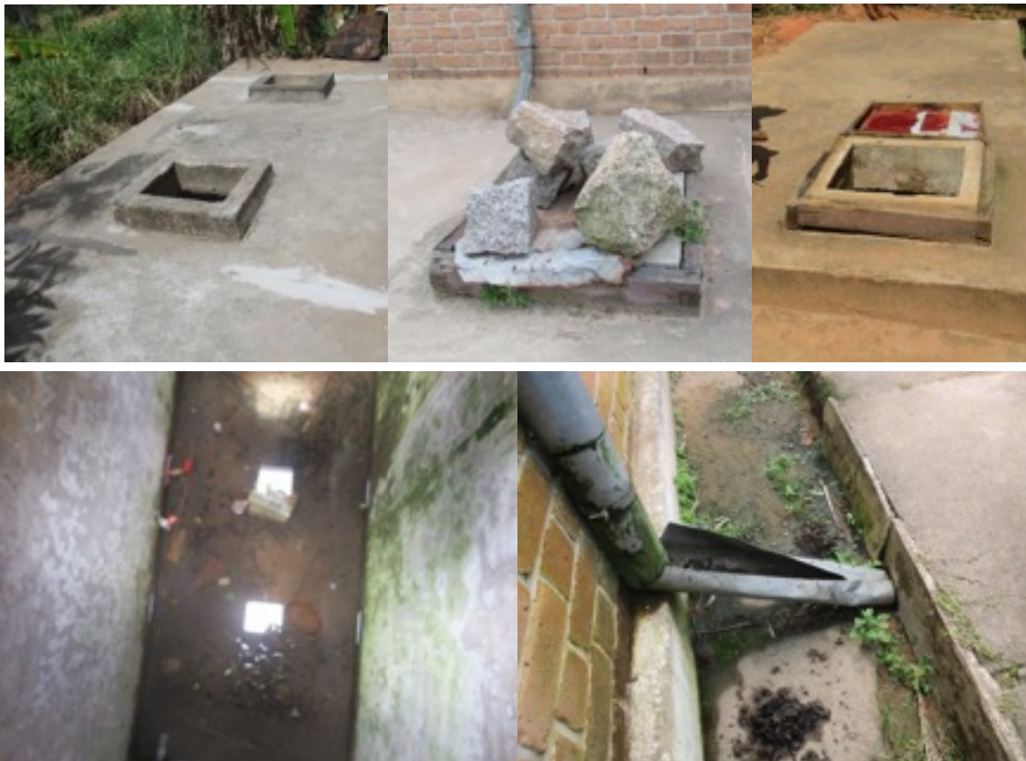
Tanks were open to contamination and much of the guttering was in a poor state.
