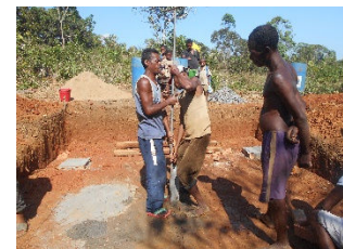
Start of drilling work
