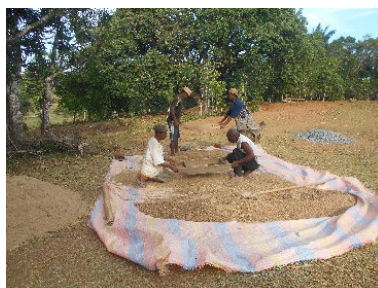
Sieving sand for the filter.
